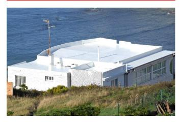
Elastic and seamless coating, weather resistant and excellent bonding. No reinforcement usually required except at critical points.
