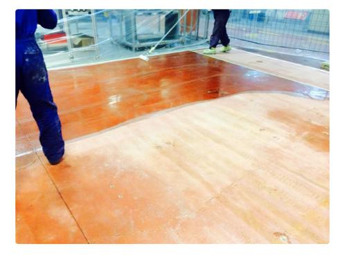
Primer based on solvent-free, two-component epoxy primer for different substrates, for both indoor and outdoor use with fast curing.
