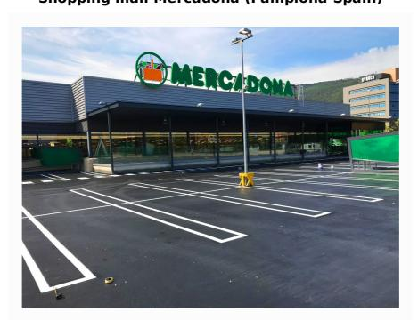
Impermax Park system (waterproofing able to resist vehicular traffic) was applied in the car park deck of the new shopping mall Mercadona (Pamplona-Spain), about 1.200 m2.
