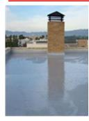
liquid waterproofing One component composition, after polymerization gives an cold-applied polyurethane membrane.
